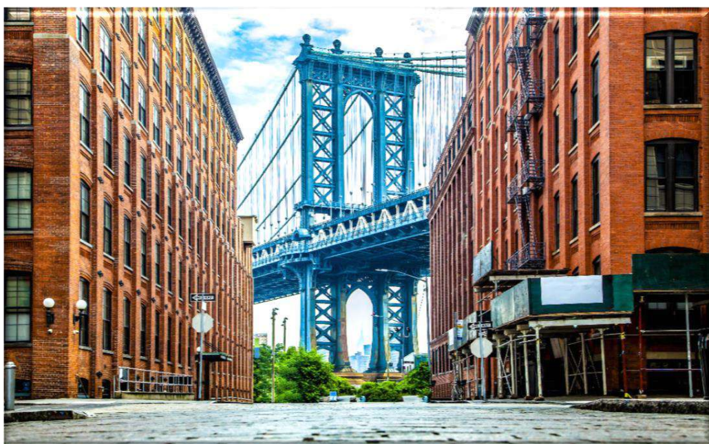
Manhattan Bridge ICSF3921D 8006449237450
